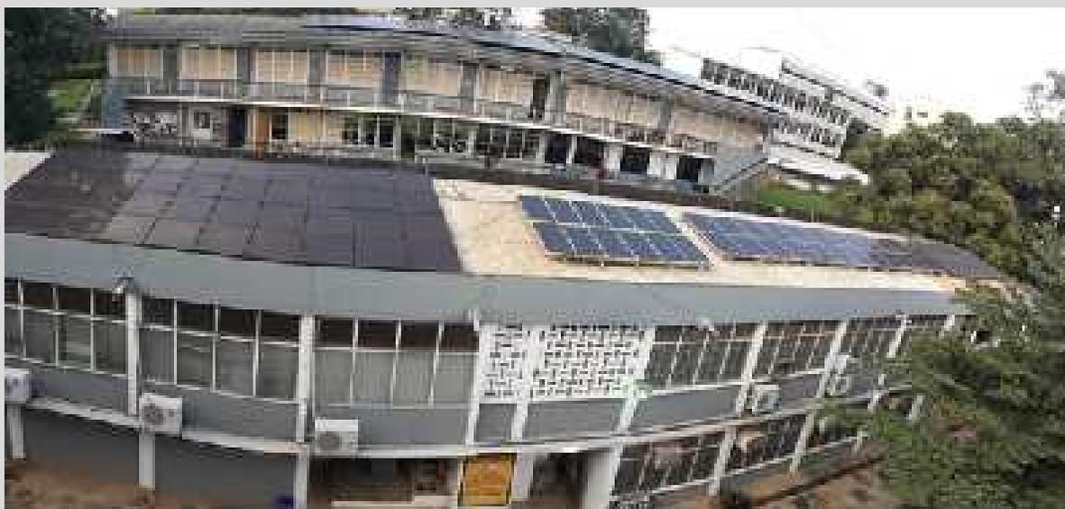
Part of the 44 kW KNUST grid connected solar PV
